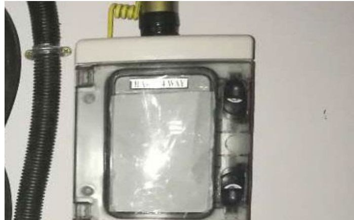
The IP rating of the distribution box does not meet the requirements
